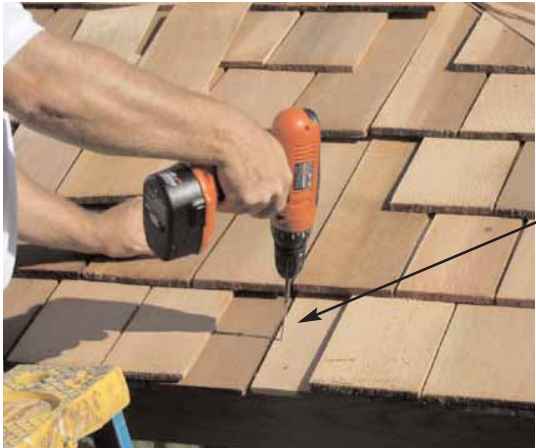
63. Where roof seams come together, secure Roof Panels to Side Rafter using 1 - 3" screw. Make sure to screw into Side Rafter
